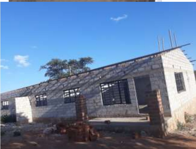
THE CONSTRUCTION OF THE HOUSE
