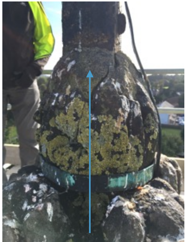
Concrete fill to the base of the iron cross
